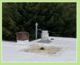
The red chimney is for the ovens, and the round metal thing is for the grill hood that was recently replaced.
